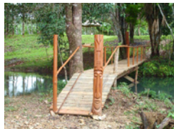
Completed bridge with ramp across the creek
