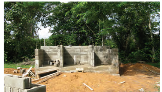
Restroom area under construction to use renewable energy sources
